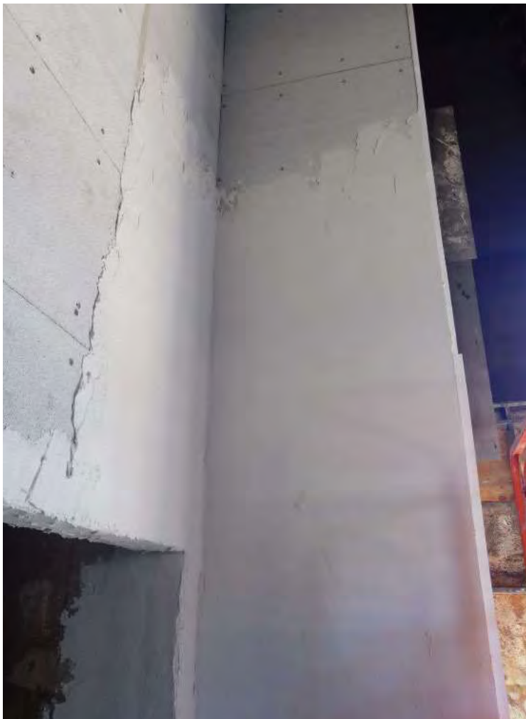
FIGURE 6: CEMENT RENDER INSTALLATION
